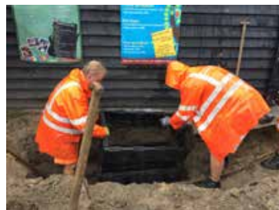
Adding layers until the height is correct.
