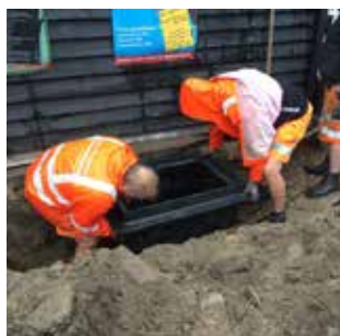
Placing the frame
