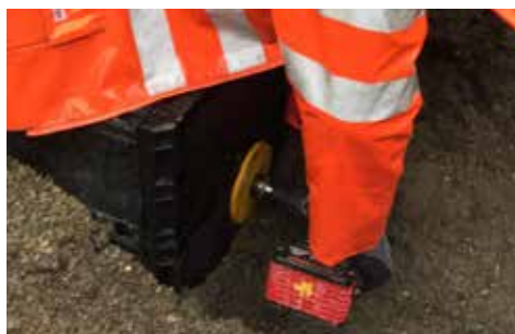
Making holes in the manhole
