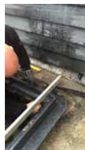
Leveling the frame before the covers are placed.
