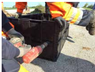
Making holes in the manhole
