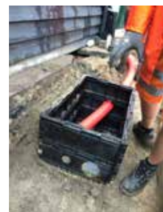
Adding layers until the height is correct.
