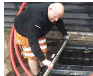
Leveling the frame before the covers are placed.
