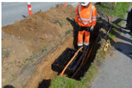
Installing first layer and base. Make sure it is level.
